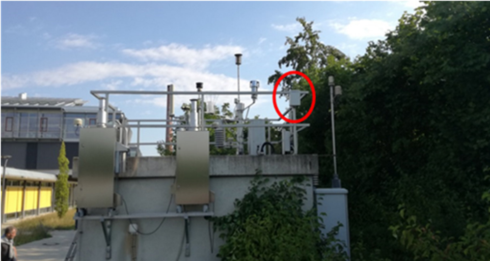
Figure 6: EDM80NEPH at the measurement site LfU headquarter
